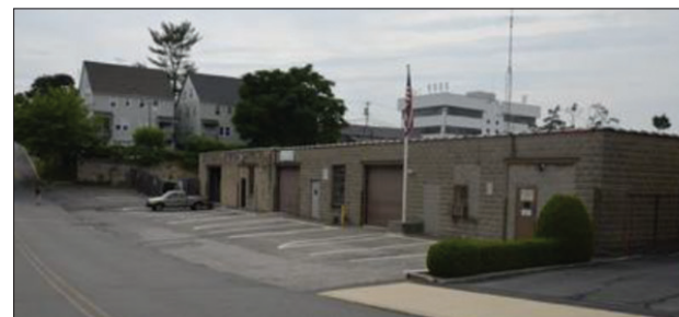
Sold to the Village of Rye Brook. The property consist of approximately 11,000 SF of building and 33,000 SF of land. NYCRG was the sole broker.
